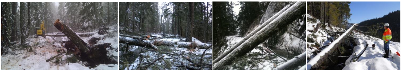
2012 Ice Storm Damage on Low Line and Farmers Canals.
